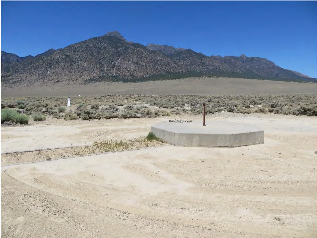
Figure A-1. Concrete Cap That Covers the UC-3 Borehole (August 2020)
